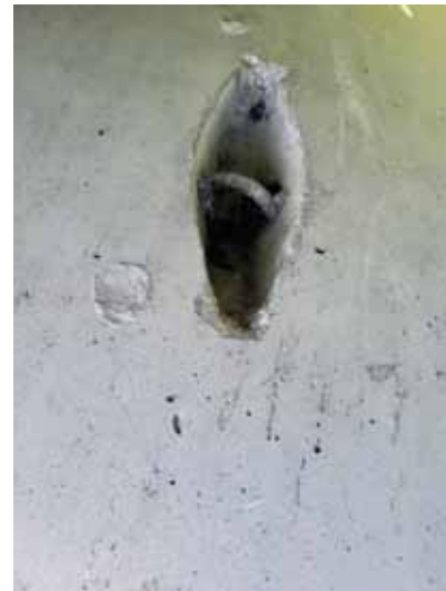
Location 16: Pipe and filter fabric was exposed. Ground cover was missing from around the pipe. Recommended sand/cement bags over and down the pipe to the toe of slope to prevent erosion. Grout lifting hooks on sides of structure.
