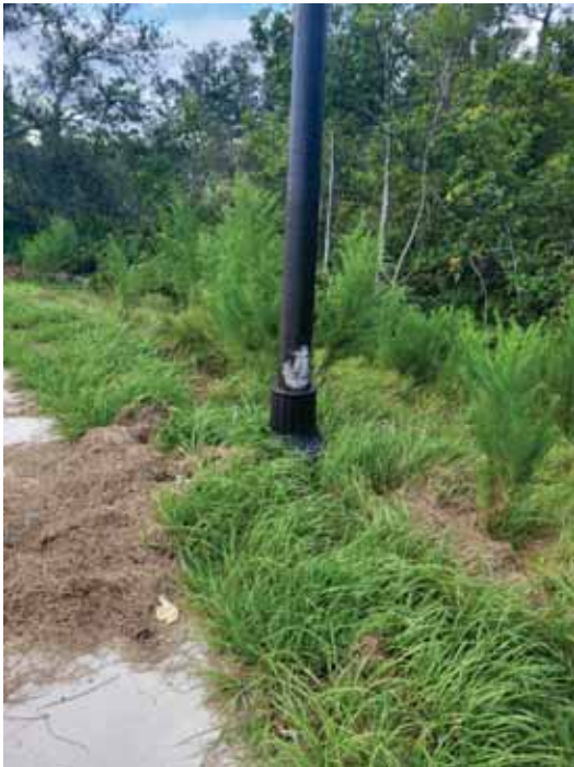
Location 16: Pipe and filter fabric was exposed. Ground cover was missing from around the pipe. Recommended sand/cement bags over and down the pipe to the toe of slope to prevent erosion. Grout lifting hooks on sides of structure.
