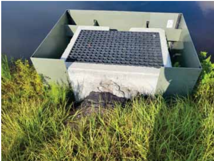
Location 16: Pipe and filter fabric was exposed. Ground cover was missing from around the pipe. Recommended sand/cement bags over and down the pipe to the toe of slope to prevent erosion. Grout lifting hooks on sides of structure.
